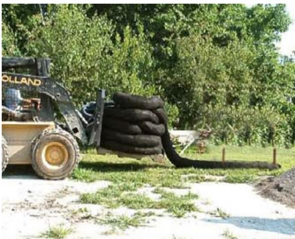
1. Position pallet and fork lift at the beginning of the area to be treated. Fork Lift will be driven backward to off-load SiltSoxx™, so be sure there are no obstructions in the path of the equipment. Have an additional safety person to spot area behind loader, if needed.
